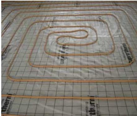
Fig. 8. A picture of heating pipes from the floor [5]
